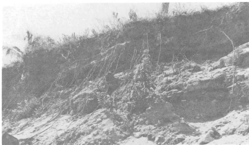
FIG. 1.—Ravages of erosion on hillsides in the Dominican Republic.
