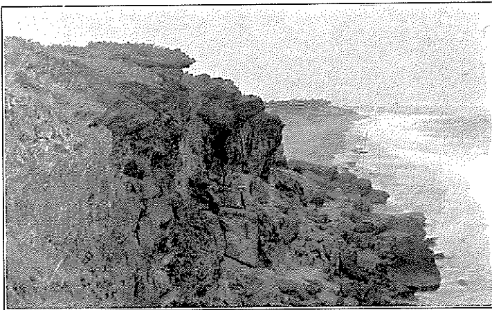
FIG. 16. Seaward face of a consolidated San Juan dune west of Arecibo, showing the undercutting by the sea and the destructive power of the wave action.
