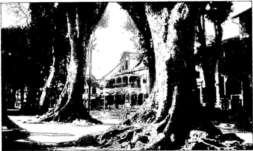
FIG. 1.—Street of Paramaribo, Dutch Guiana, lined with trees of West Indian mahogany. (Original).
