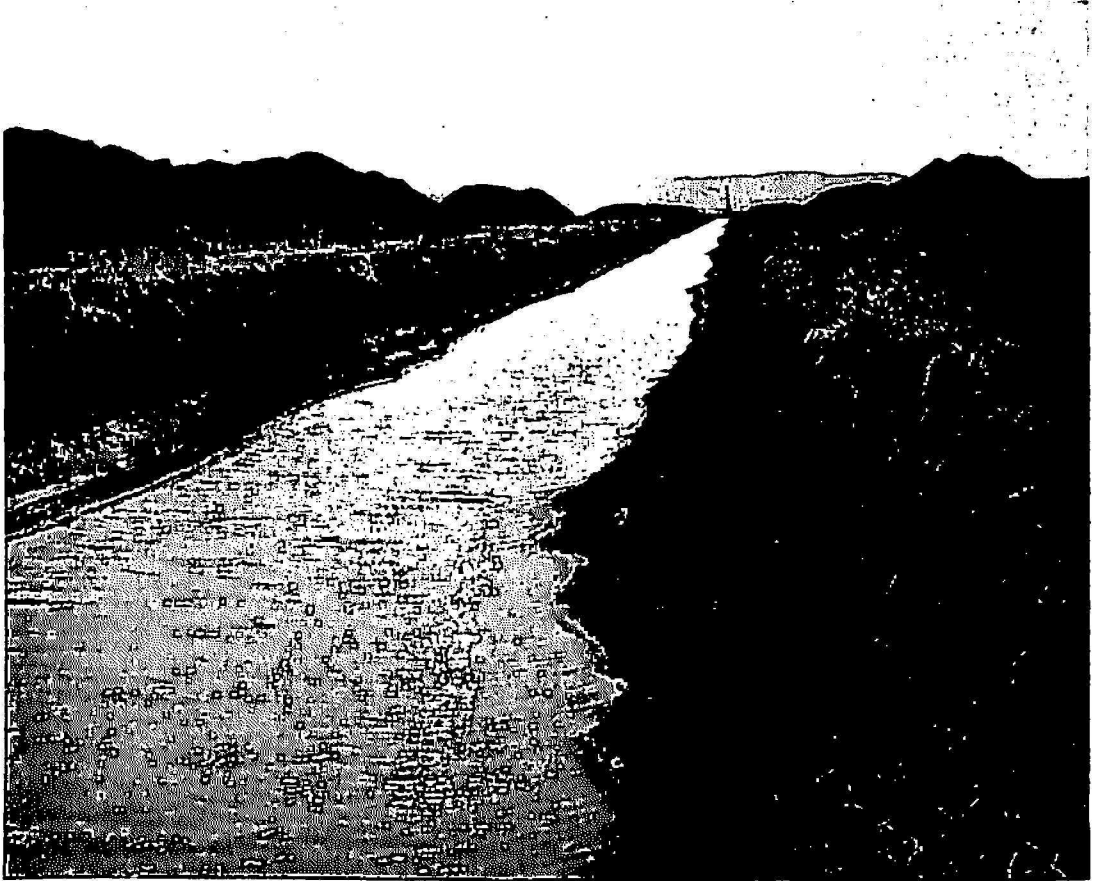
FIG. 4—Part of main southern drainage canal in Lajas Valley.
