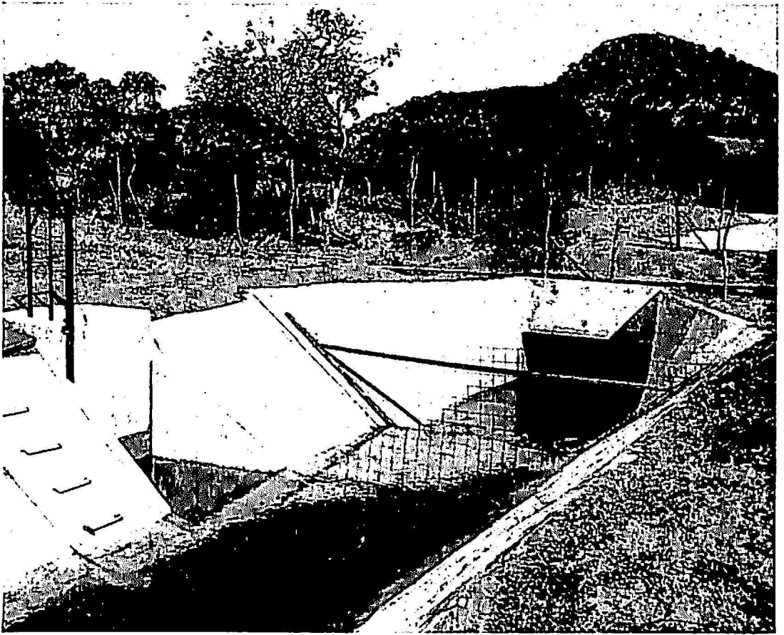
FIG. 3—Part of main northern irrigation canal with gate at the side; Lajas Valley.
