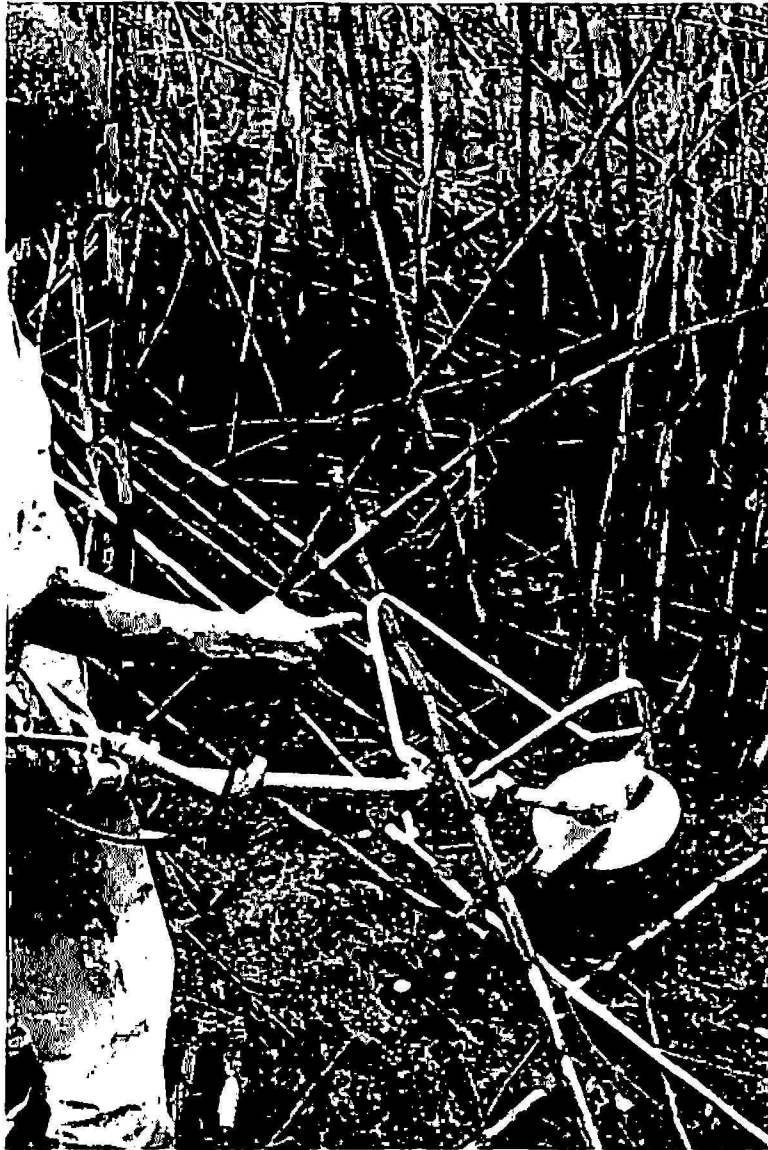
FIG. 3.—An unsuccessful attempt at windrowing by the use of diversion bars. Note the cane stalk that has tangled.
