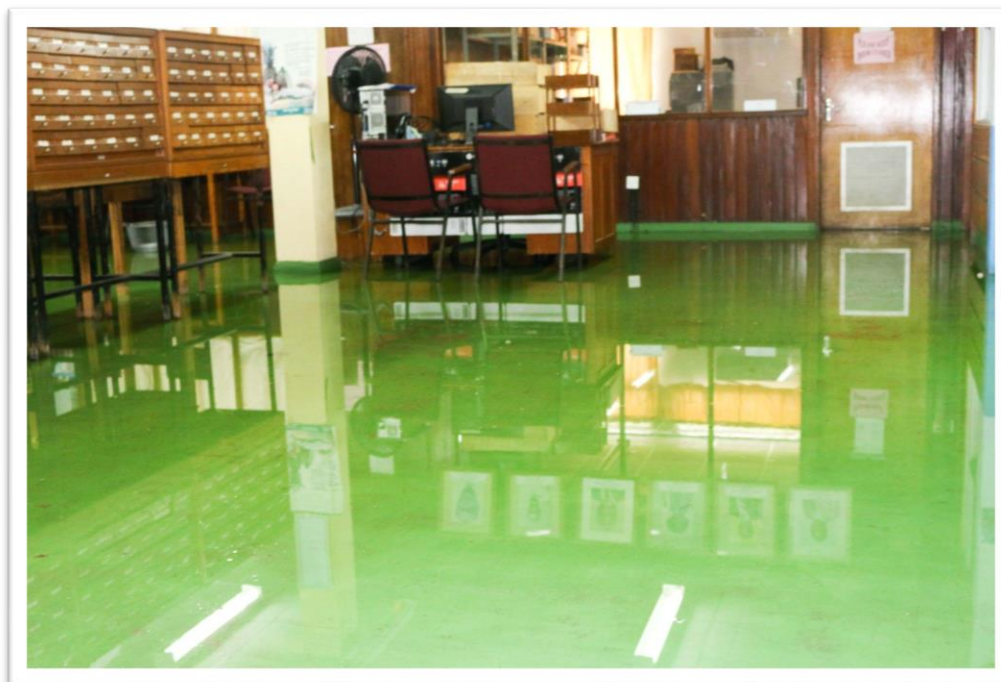
UG Library Ground Floor - 2017 Flood
